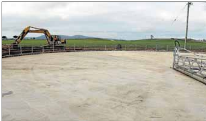
The curved yard features a water-driven backing gate that cleans the yard as it moves behind the cows.
