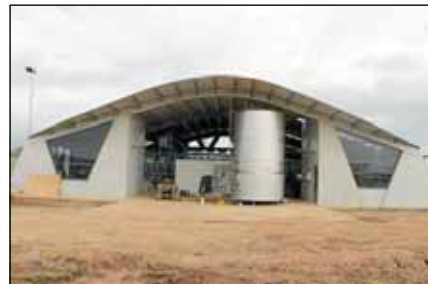
The dairy with its huge curved sweeping roof that improves ventilation.
