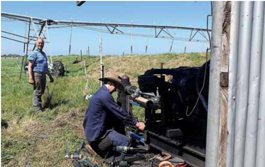
Trevor and Jono Porter installing the pump equipment. Jono, a fitter and turner, is installing a drive shaft in the irrigation pump. Photo by Clare Porter.
