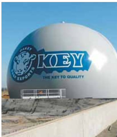
The Oakey plant is designed to produce biogas (primarily methane) which is stored for use in a 6000m 3 flexible PVC-coated polyester storage balloon.
