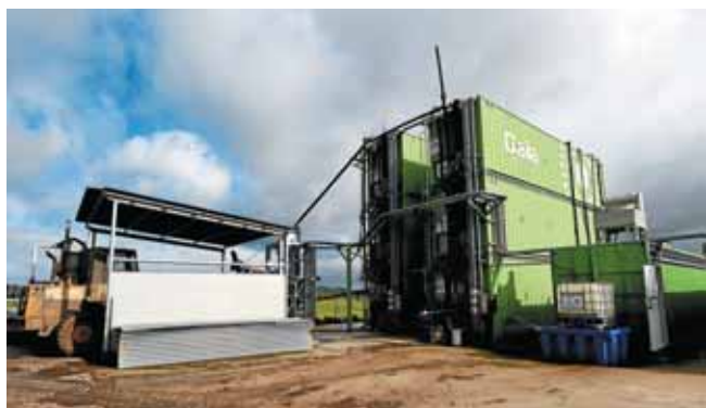
Manure is first processed in the shed on the left — solid waste is collected and spread over paddocks as fertiliser, while everything else is fed to biodigesters in the Gaia system to produce electricity.
